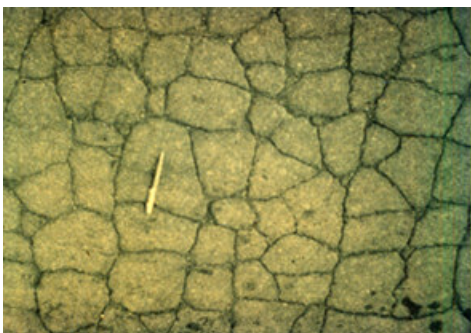
Figure 2.1: Example of asphalt pavement where reinforcement could provide a benefit
