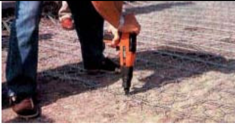
Figure 7.5: Fixing of steel mesh grids
