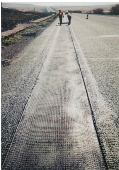
Figure 7.2: Glass fibre grid placed on levelling layer prior paving
