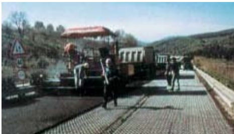
Figure 7.7: Final paving operations
