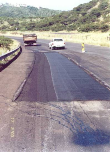
Figure 7.1: Placed, tacked and saturated ARI prior to paving
