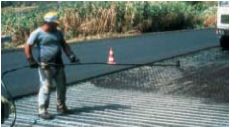
Figure 7.6: Applying tack coat prior to paving
