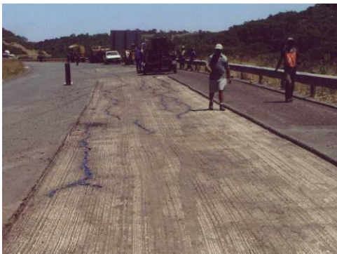
Figure 3.1: Milled surface prior to placing of ARI
