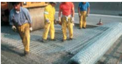
Figure 7.4: Placing of steel mesh grids on prepared surface
