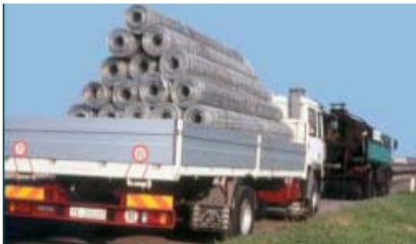
Figure 7.3: Delivery of steel mesh grids to site
